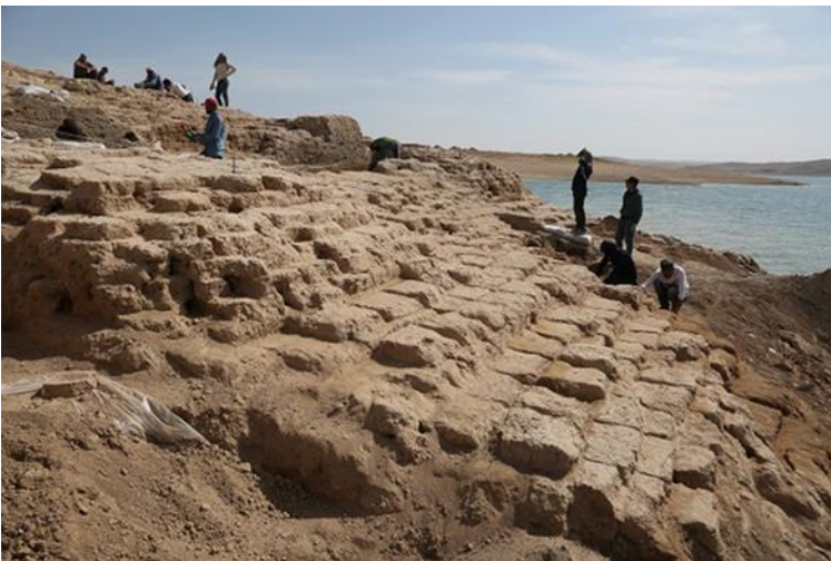
Terrace wall on the western side of Kemune Palace; photo: University of Tübingen and Kurdistan Archaeology Organization
